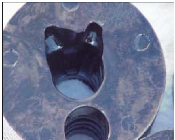
Close up of a Degraded Grid.
